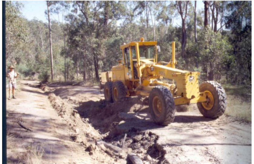
Figure 5. - Grader repairing track and installing drains
