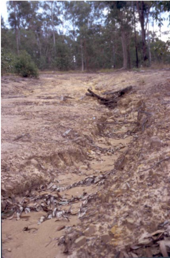
Figure 4. Badly eroded access track
