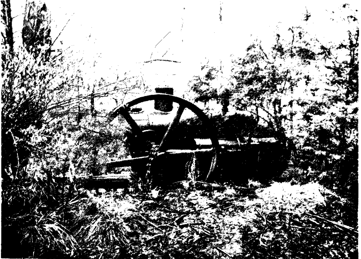
Figure 1 Substantially intact 12" bore by 24" stroke steam engine which powered a logging winch at the No.4 mill - an unusual and not very successful application for this type of engine. Photo: Peter Evans.
